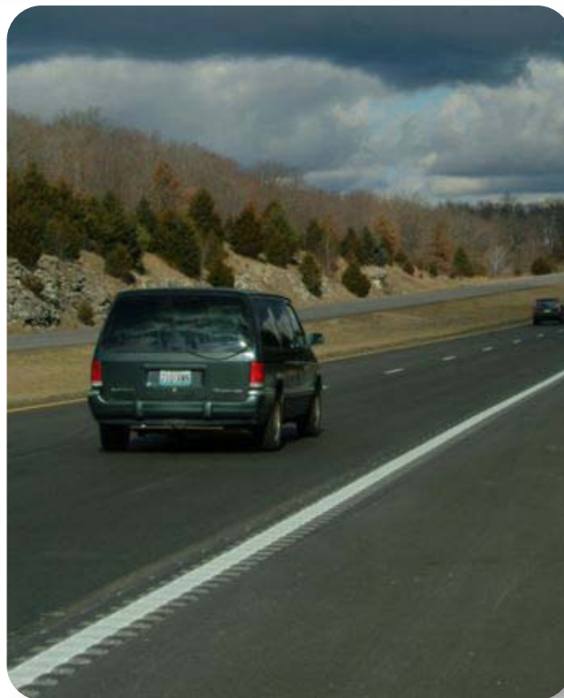
Edgeline Rumble Strips
